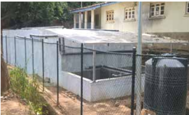
Sewerage treatment plant
