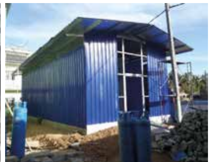
On Midway of construction 2017
